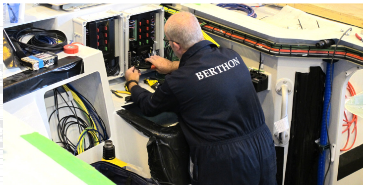
(4) FITTING THE HULL ELECTRONICS
