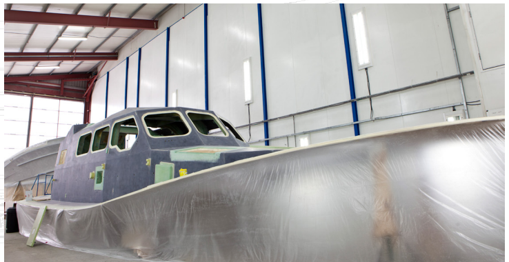
(3) DECK & WHEELHOUSE MOULD READY FOR PAINTING
