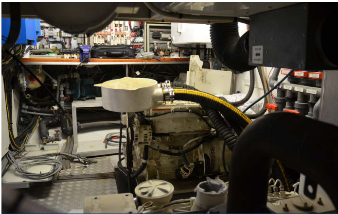
ORIGINAL ENGINE ROOM
