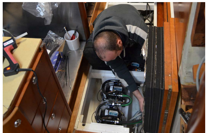
NEW REFRIGERATION COMPRESSORS
