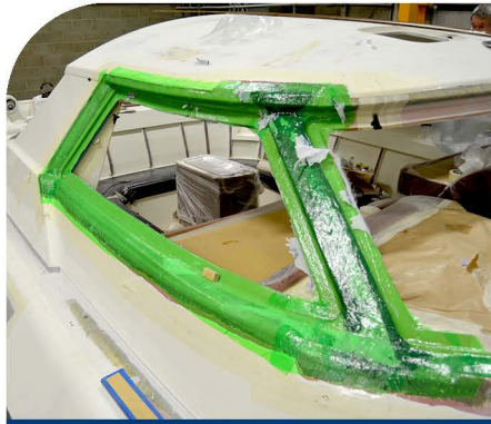
REPAIRING CRACKED MULLIONS
