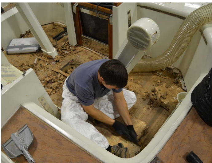
REMOVING THE OLD TEAK DECK
