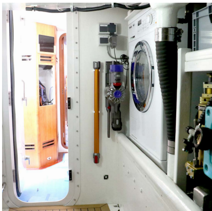
NEW WASHING MACHINE FITTED IN LAZARETTE
