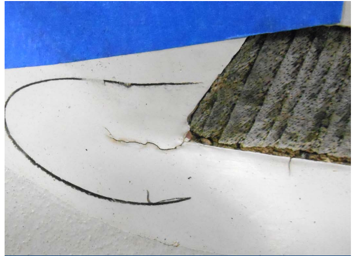
CRACKS ON THE MULLIONS
