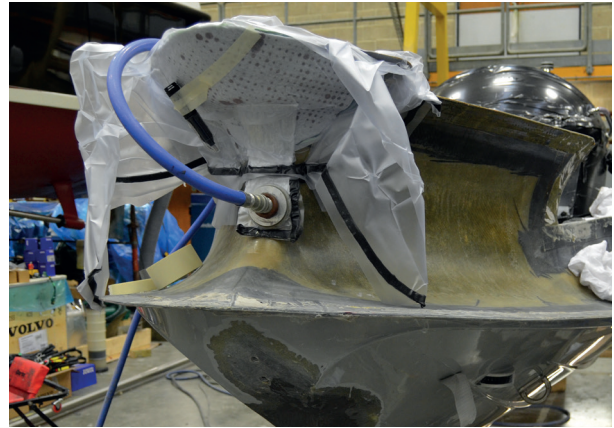
Consolidation of carbon repair
