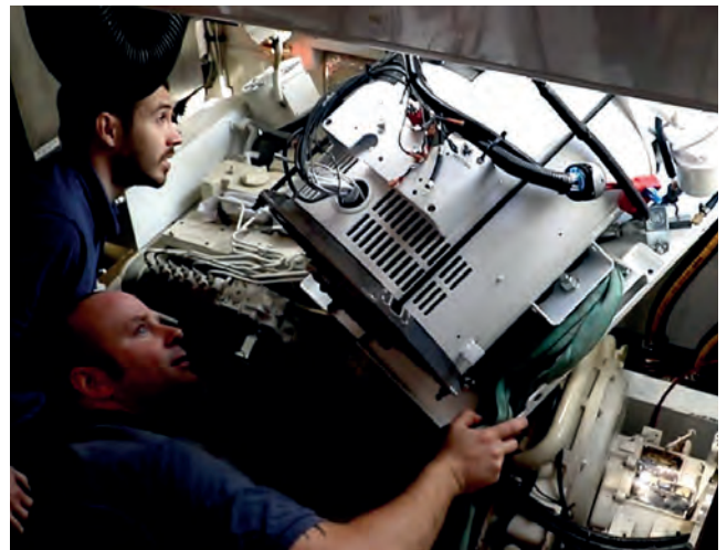
Installing the new Kohler generator
