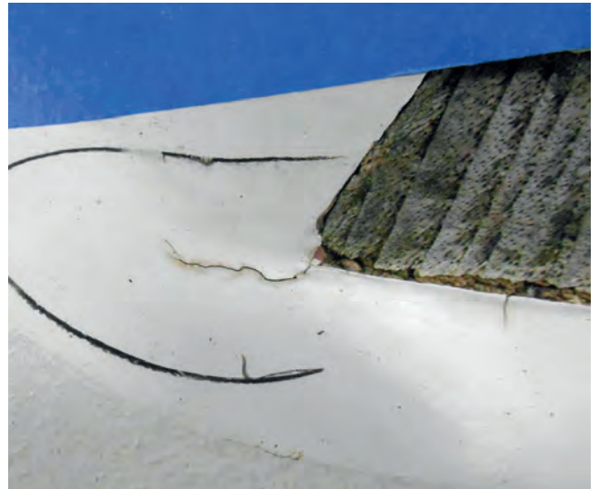
Cracks on the mullions
