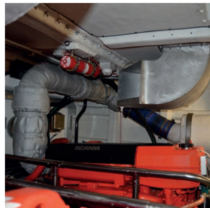
New ducting and engine
