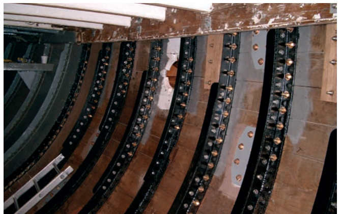
Repaired and replaced ribs
