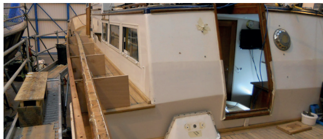
New teak laid
