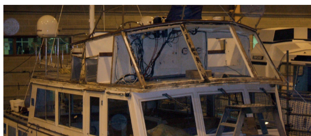
Removing rotten wood from flybridge and superstructure
