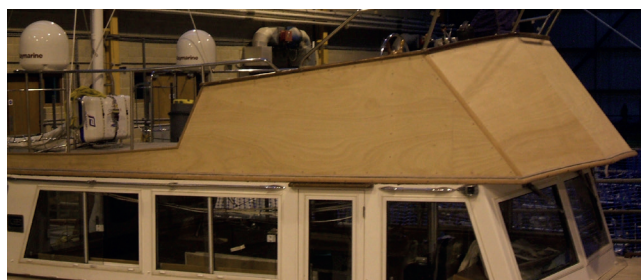
Rebuilt flybridge and superstructure
