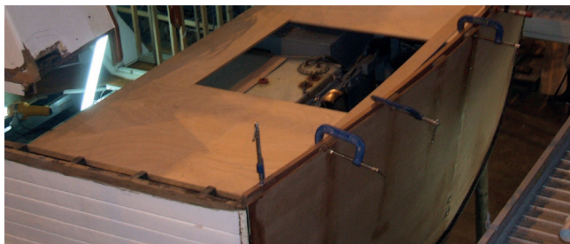
Rebuilding the transom
